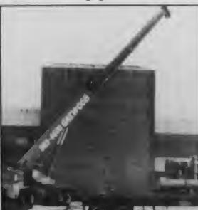
Cranes were needed to move the massive air conditioning unit onto Building I.
