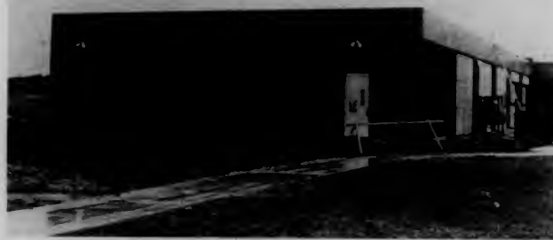
As of April 1, "U" Building will open its doors to the Physical Ed. Dept. and students. The temporary facility is 160 feet in length and 50 feet in width. (Photo by Donn Lynan.)
