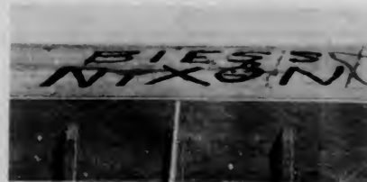
The words of the common man were voiced and viewed as seen atop a roof at Harper; workers laying a new roof put down their message loud and clear...
