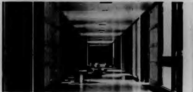
New music wing in final stage of construction. (Photo by Ken Kissam)
